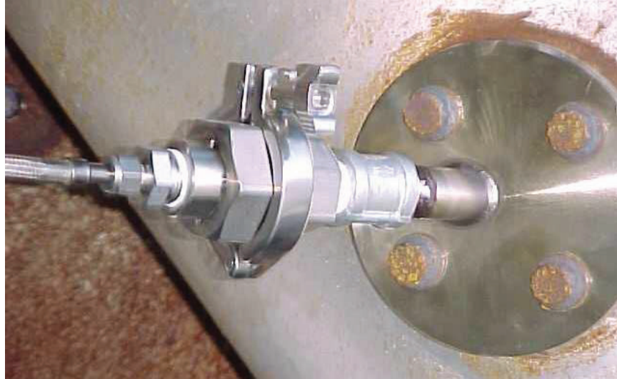
Figure 3 Frame FSA Installation Primary Zone
